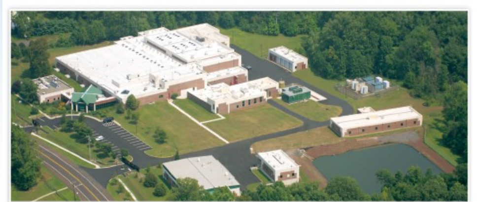
Above: Forest Park Water Treatment Plant in Chalfont, PA
